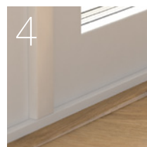
4 End moulding Finishing up to threshold, sliding doors, etc.
